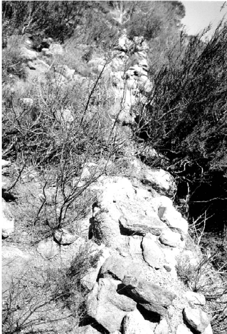
Fig. 11. Southern section of perimeter wall.
