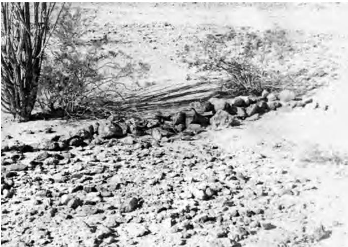
Figure 11. Large retaining wall; note silt buildup.
