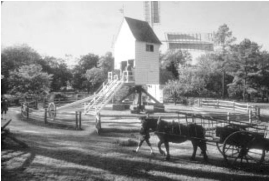
Fig. 11. North European wooden post mill of the type familiar in New England and Russia. The entire mill body could rotate 360 degrees to take advantage of shifting winds. This example is reconstructed in Colonial Williamsburg.
