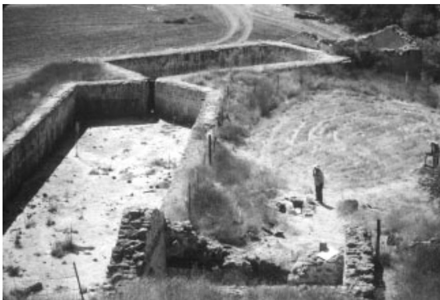
Fig. 9. The Santa Inés mill complex, built in 1820-23, consisted of a fulling mill (lower right, 1822-1823), a large reservoir (left), a small reservoir (upper center), and a grist mill (upper right). The complex was powered by water directed through a ditch two miles in length.
