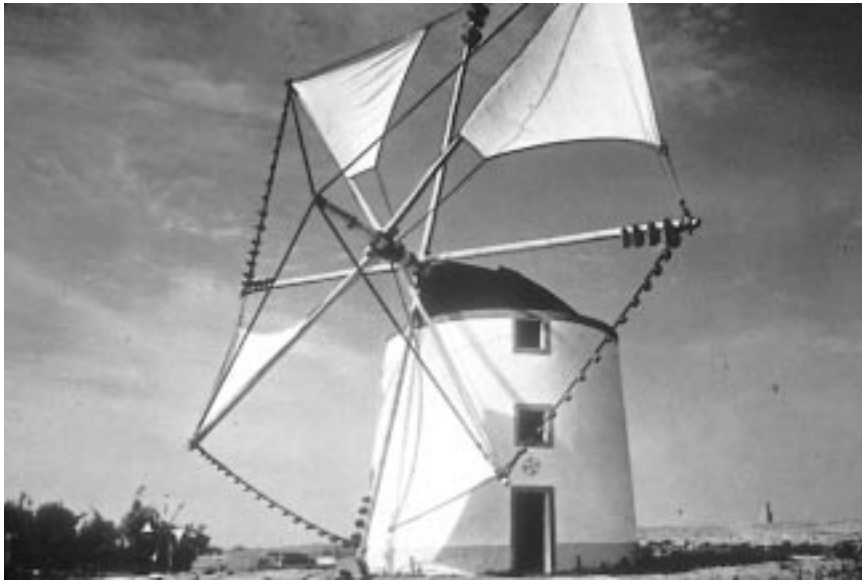
Fig. 10. Mediterranean style windmills consisted of massive stationary towers of masonry. Only the cap and blades of the windmill could be rotated. This example is from Portugal.
